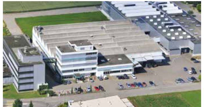
The site in Seon is a competence centre for Fehlmann AG in every respect: Development, planning, production and administration are housed here.
