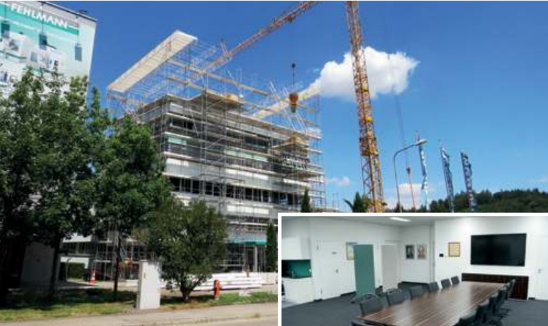
Renovation of the facade on the south side.
